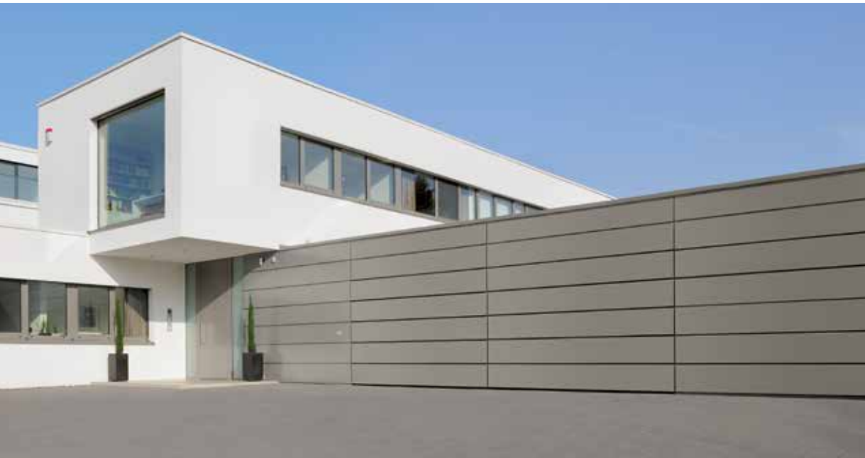
On-site cladding with aluminium compound board
